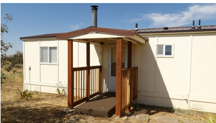
The porch is made of pressure treated timbers with spindles of red wood. The ramp was repaired and now has a new brown indoor/outdoor carpet.
