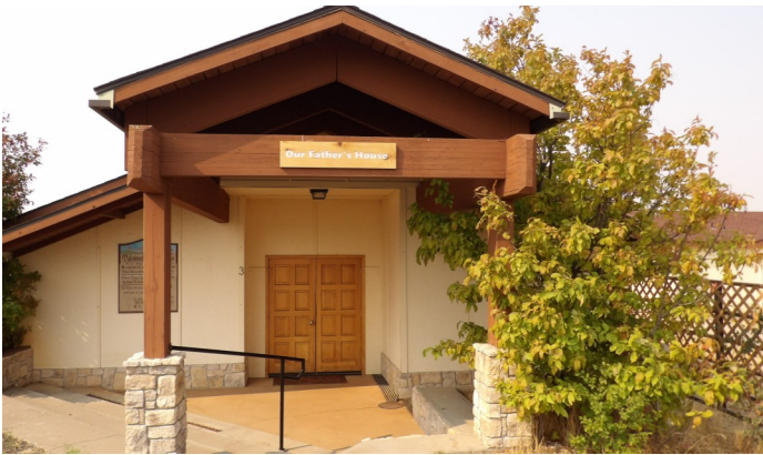
DOOR above is that into Our Father's House, the chapel at Marymount Hermitage. [Photos 8-6-2026]
